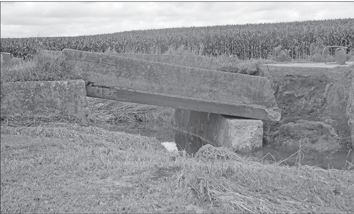
This bridge is on a private drive just south of Lena on Hwy 73. The footings are completely washed away.
